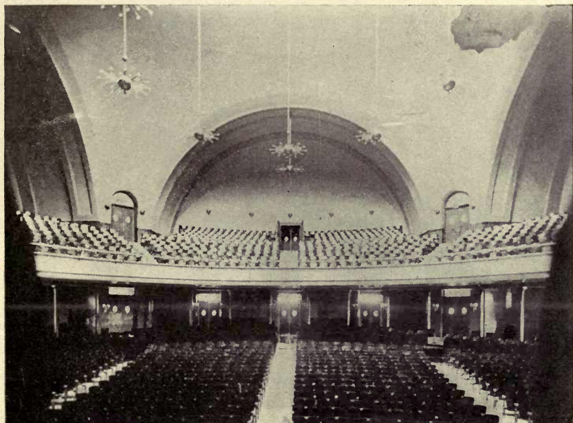
FIG. 6. PHOTOGRAPH SHOWING AUDITORIUM BEFORE CHANGES WERE MADE
